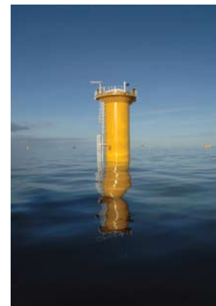
Steel monopile foundation
