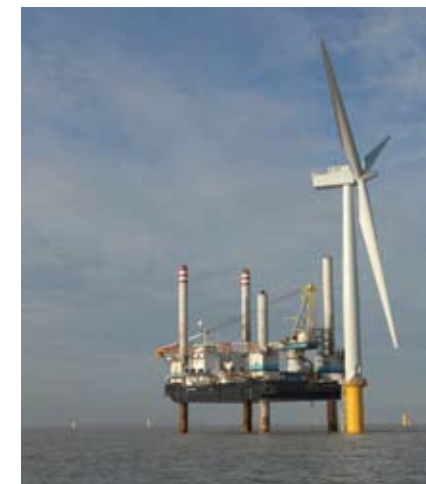
Construction vessel and turbine
