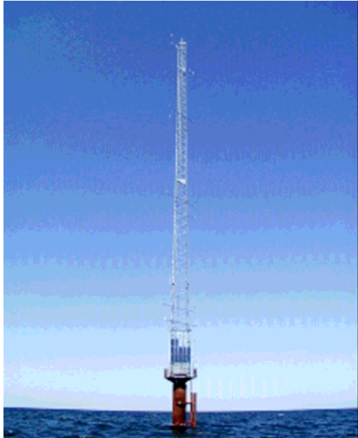
Figure 1 Offshore met station with boat landing arrangement
