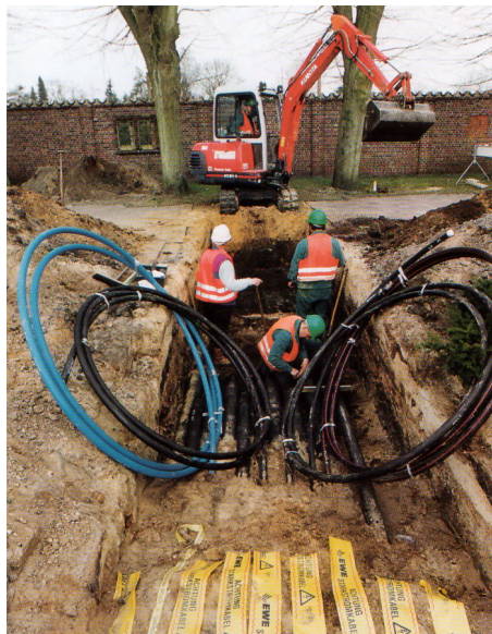
Figure 8.4: Typical trench construction
